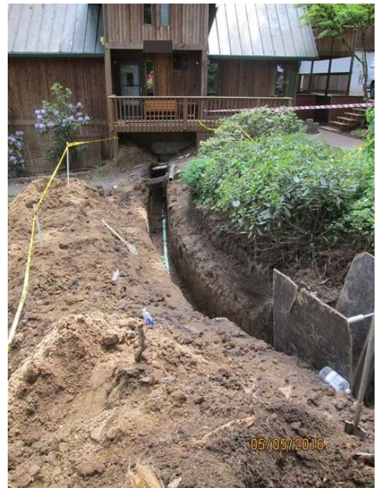
Figure 3. View of trench work area in front of house
